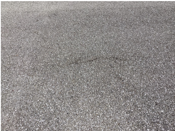
Pavement cracks
