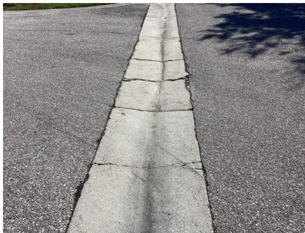
Gutter cracks
