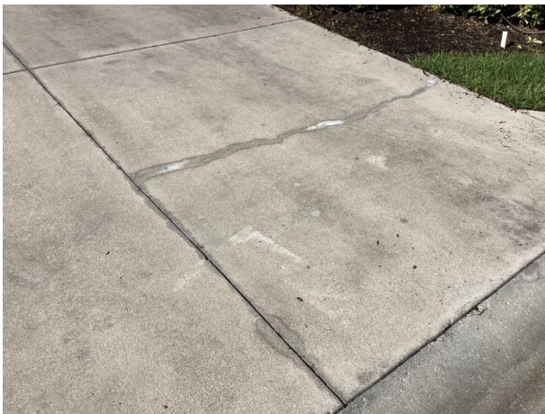
Driveway cracks
