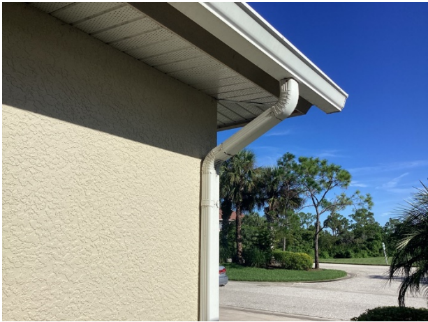
Aluminum gutters and downspouts
