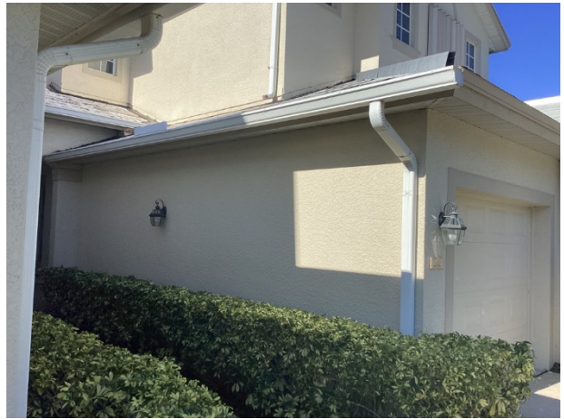
Aluminum gutters and downspouts
