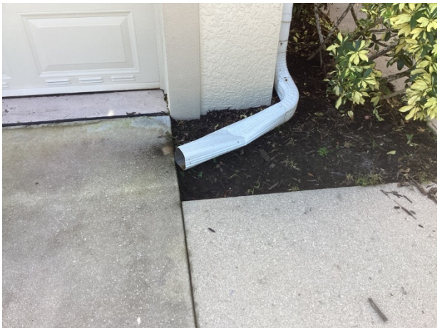
Dented downspout
