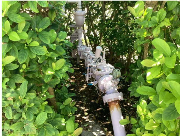
Water main shutoff valve
